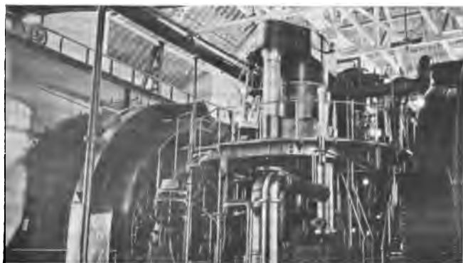
C. ONE OF THE CALUMET AND HECLA HOISTING ENGINES.]
